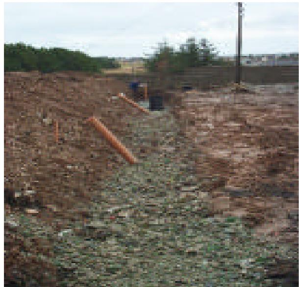
**Plate 3. Clay soil** trench has to be dug a lot deeper, 18", usually with lateral drains, filled 2/3 with glass then clean stones.
