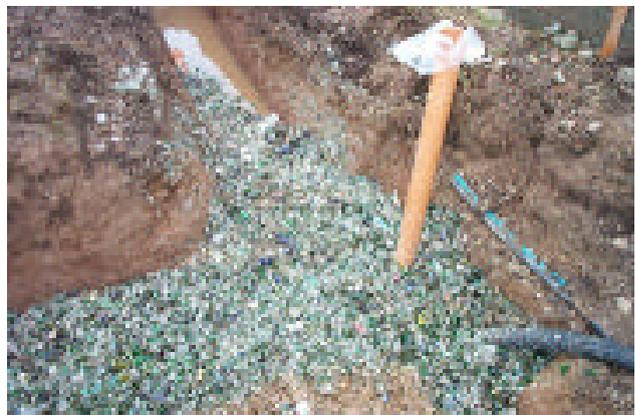
For both soil types drains have to be dug at an angle (downwards) have to make sure there are no uneven dips or hollows in the descent as water will eventually
